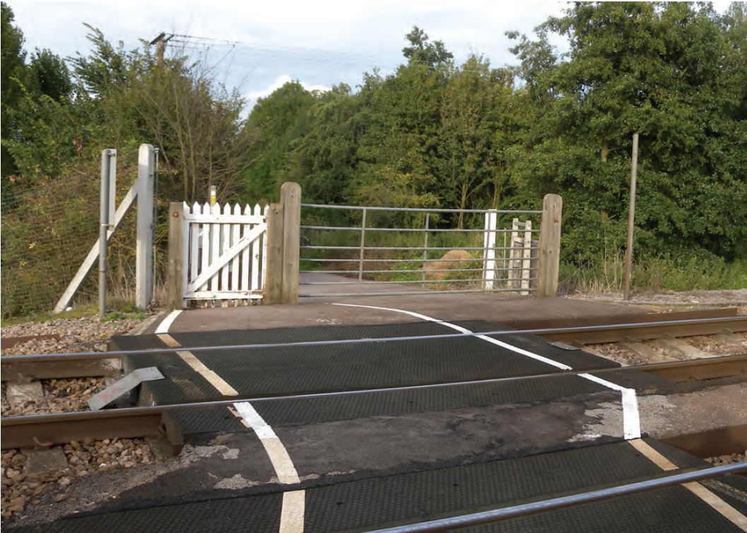
Gipsy Lane level crossing, Needham Market, Suffolk. The private road crossing has been closed by agreement between Network Rail and the beneficiary. The public footpath crossing remains in use. Credit: Rail Accident Investigation Branch.
