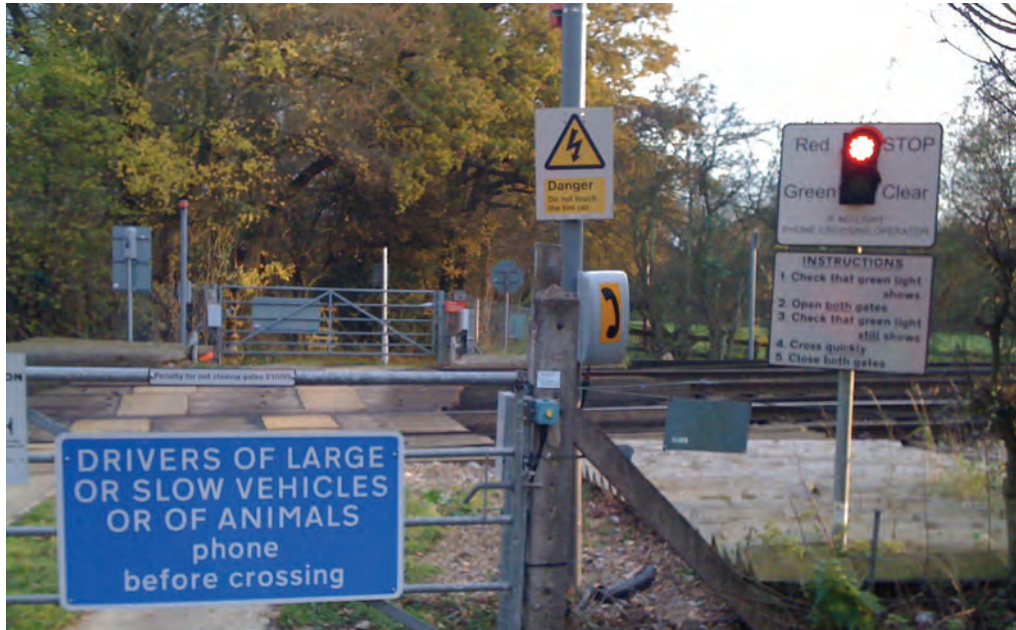
Lower Pratts private road level crossing in West Sussex. This crossing was previously controlled by a telephone to the signal box, but has been upgraded to use remote-controlled gates and miniature warning lights, controlled from the signal box. Locally monitored CCTV has also been fitted. Credit: Ashleigh Keall.
