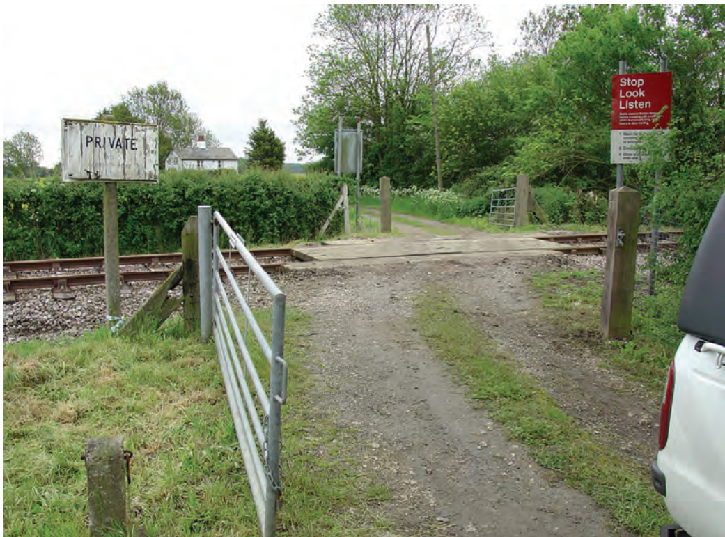
User-worked crossing on a private road at Bratts House on the freight only Saxmundham to Sizewell line in Suffolk. Note the absence of telephones or other warning devices, so that the user has to judge whether it is safe to cross by looking out for approaching trains. Credit: Rail Accident Investigation Branch.
