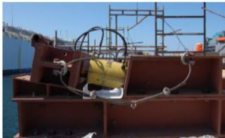
(c) Cross-Beam and Hydraulic Jacks at 11°
